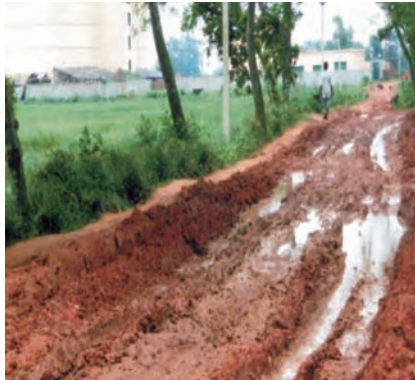
Village road - before
