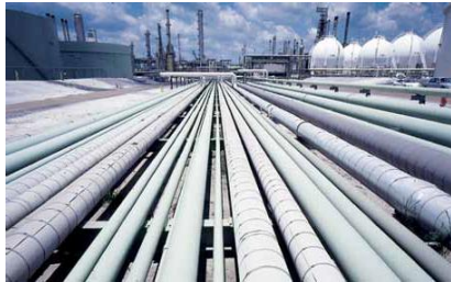
Anti Corrosive Material
